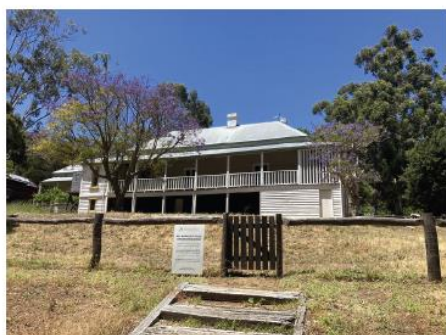
Mill Manager's House as viewed from trail
