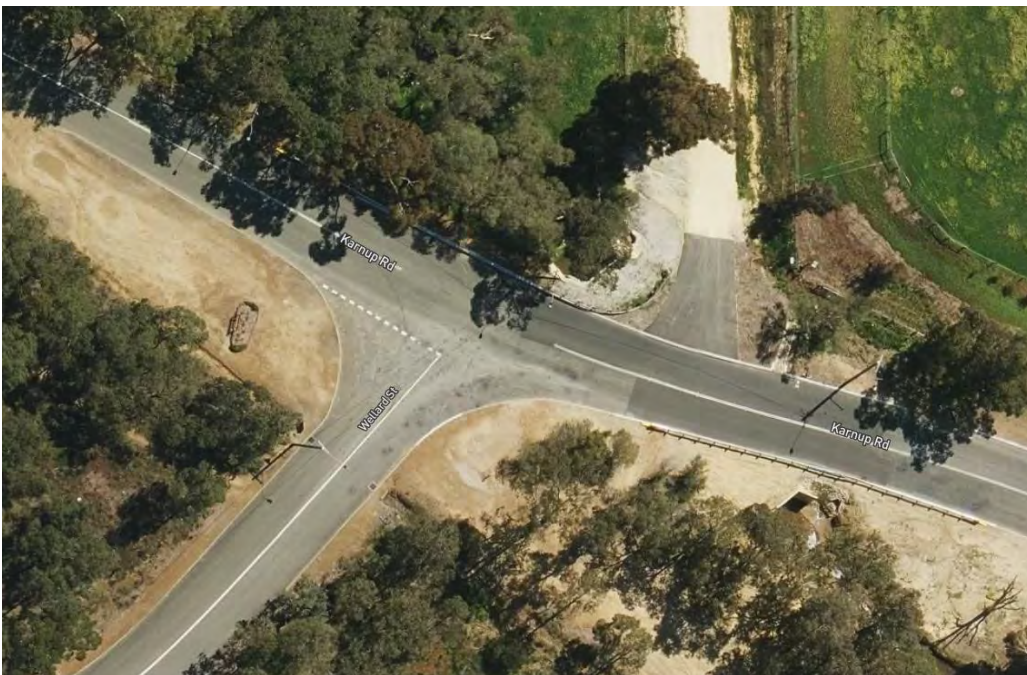
Figure 2-8 Karnup Road/ Wellard Street
