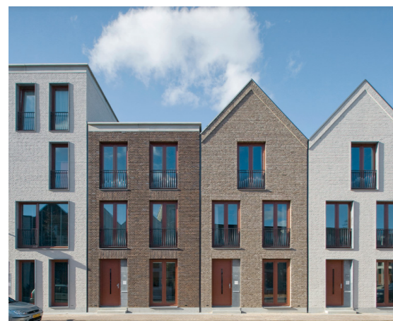
Building articulation for residential area
