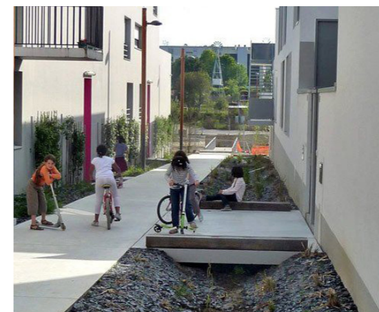
Stormwater management integrated into residential development
