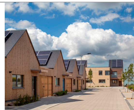
Lane access to solar powered garages
