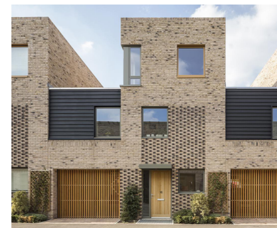
Building materials and articulation
