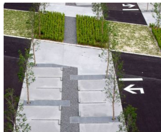
Stormwater management integrated into car parking
