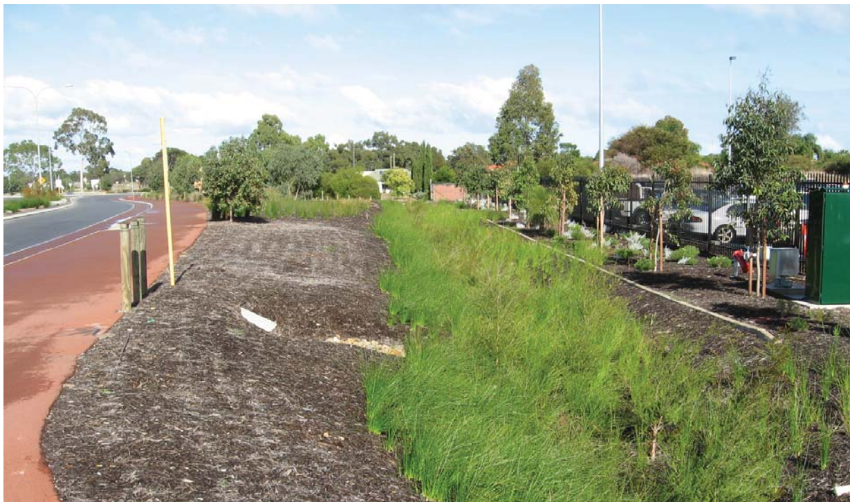
Bio Swale Example - Perth Airport
