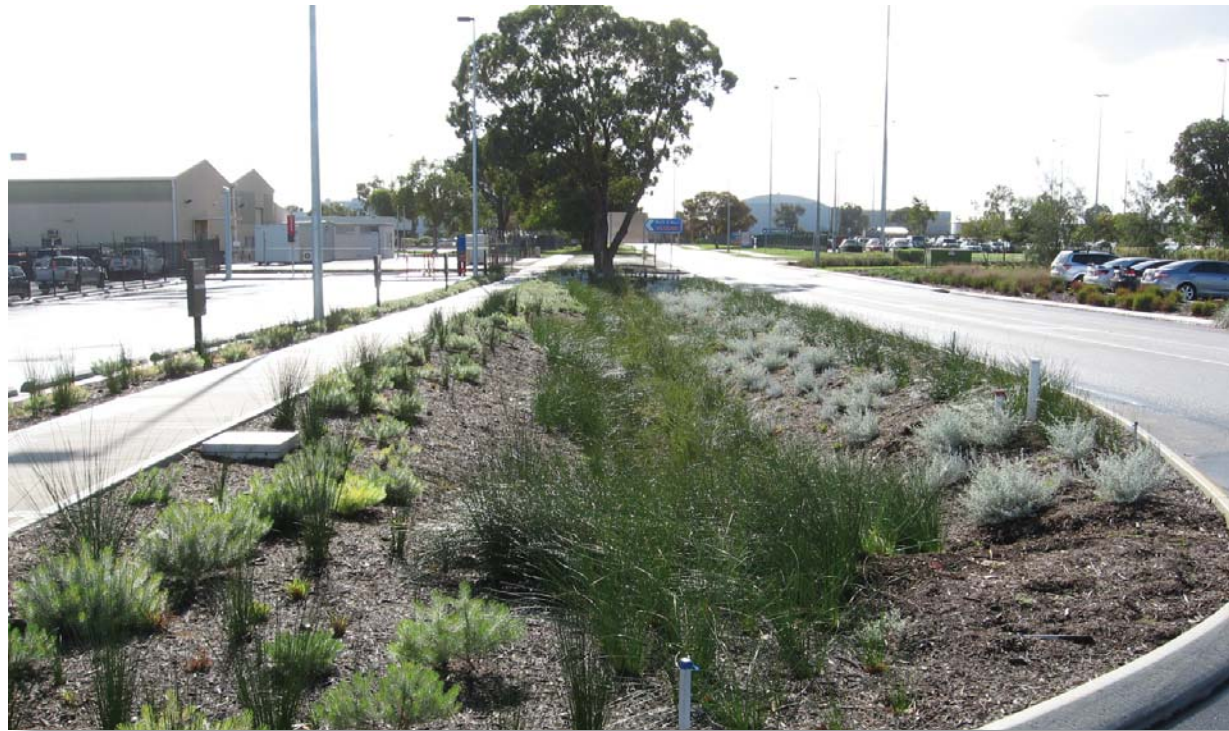
Bio Swale Example - Perth Airport
