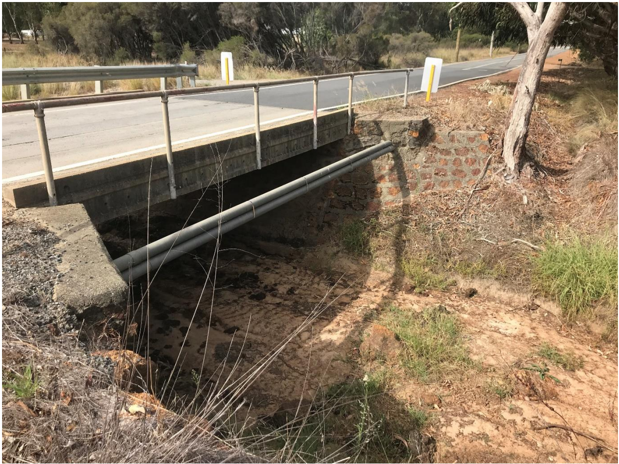
Structure No 53: Site 1.9 – Oaklands Drain at Orton Road
