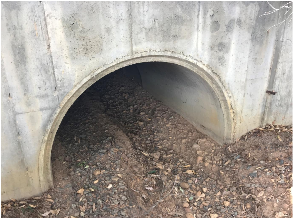
Structure No 95: Site 2.8 – Norman Drain at Soldiers Road
