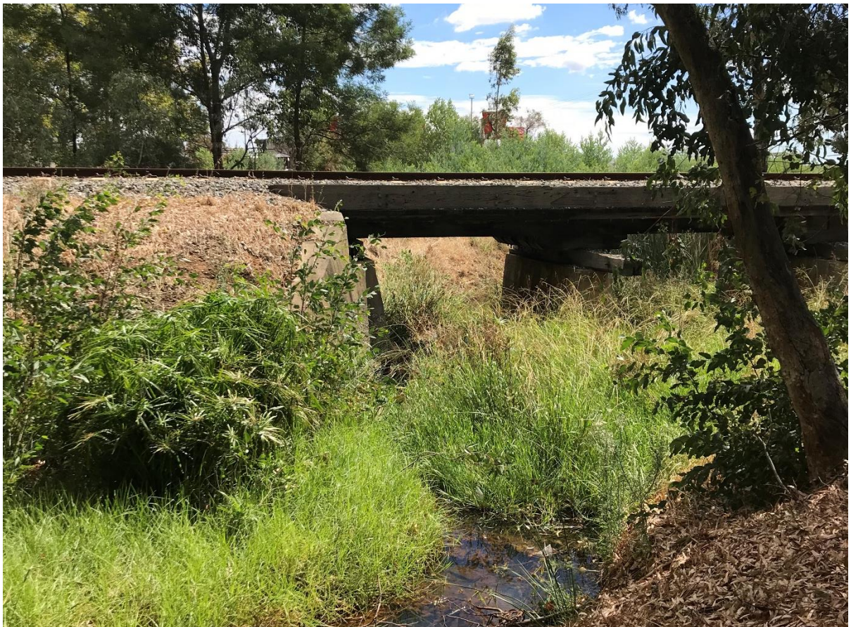
Structure No 40: Site 1.2 – Beenyup Brook at Railway
