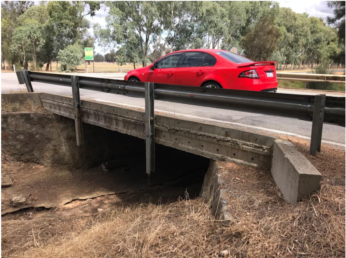
Structure No 81: Site 1.7 – Birrega Subdrain at Abernethy Road, Kargofich Road Intersection
