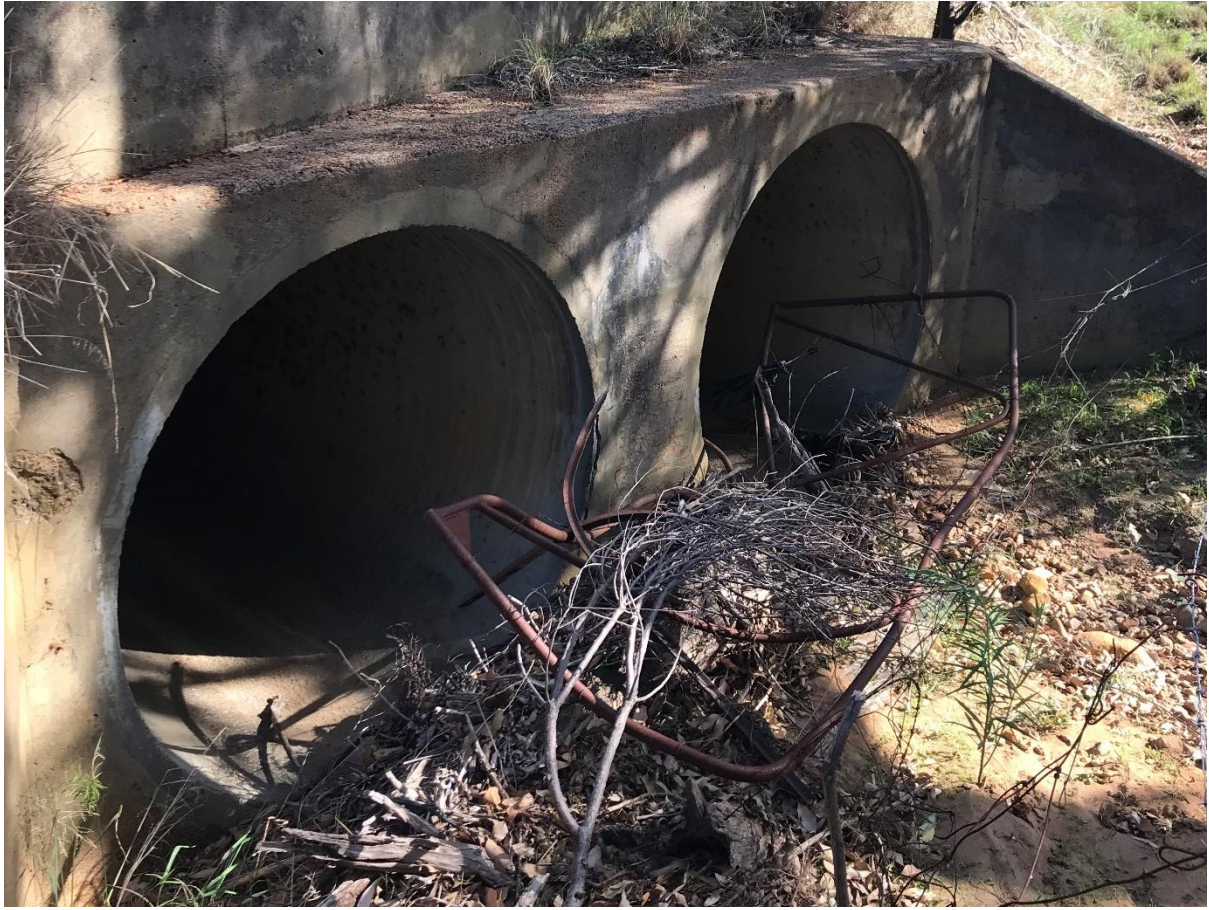
Structure No 92: Site 2.9 – Norman Drain at South West Highway
