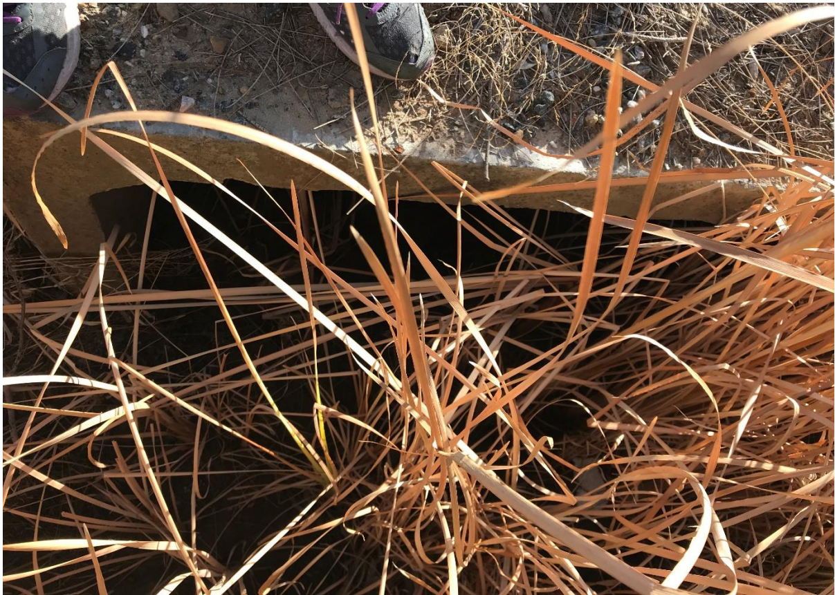
Structure No 84: Site 2.1 – Rowley Road at Darling Downs
