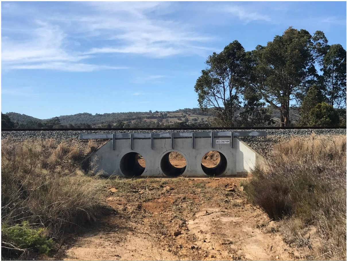
Structure No 86: Site 2.10 – Cardup Drain at Railway
