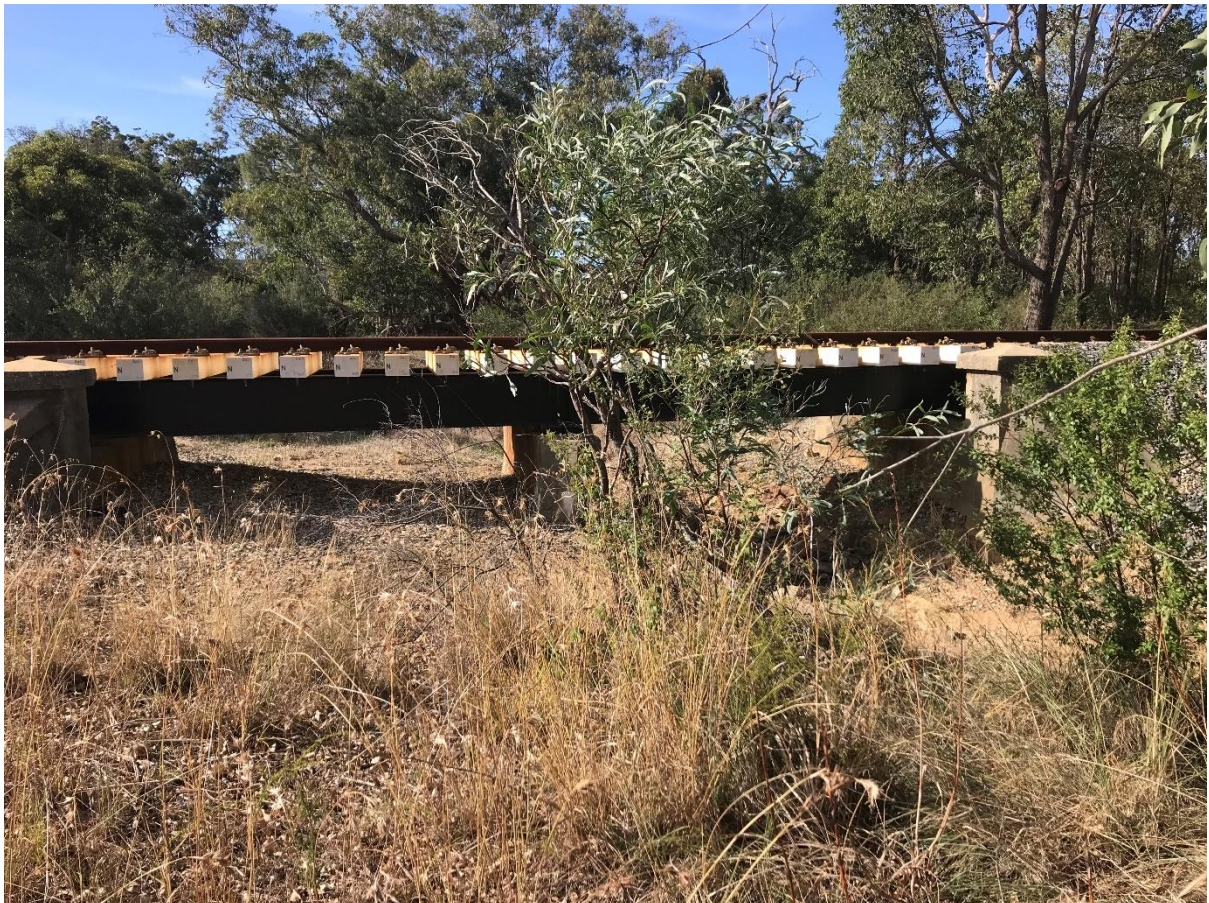
Structure No 93: Site 2.8 – Norman Drain at Railway
