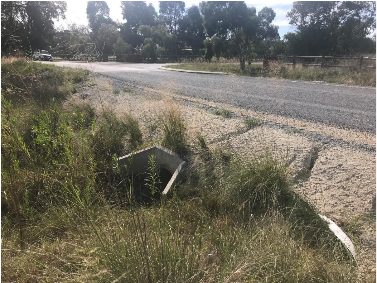
Structure No 90: Site 2.13 – Cardup Drain at Baigup Loop
