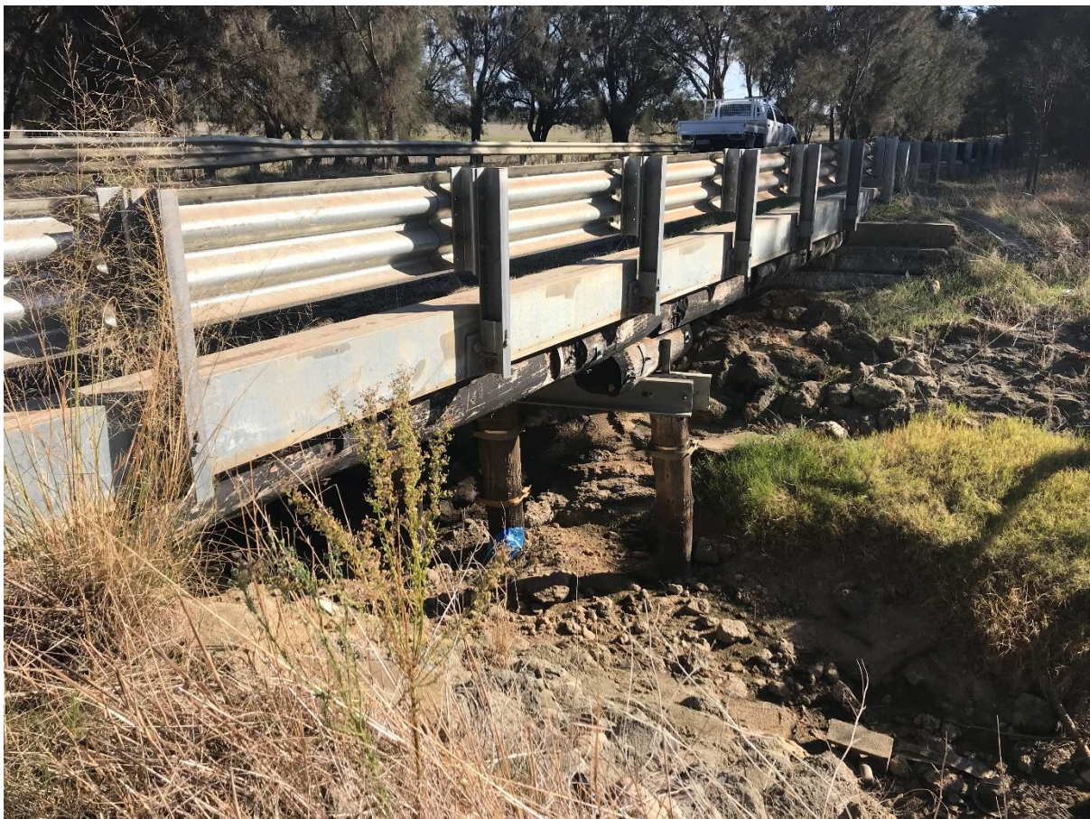
Structure No 84: Site 2.2 – Oaklands Drain at Kargotich Road
