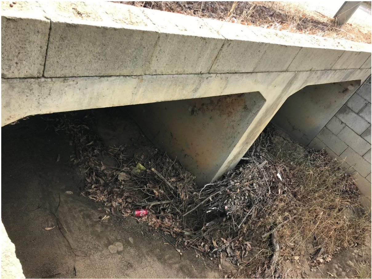
Structure No 80: Site 1.25 – Cardup Brook at Hopkinson Road
