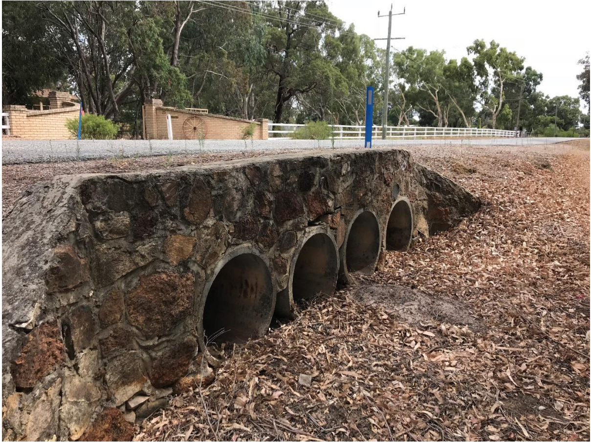
Structure No 7: Site 1.21 – Birrega Drain at Masters Road
