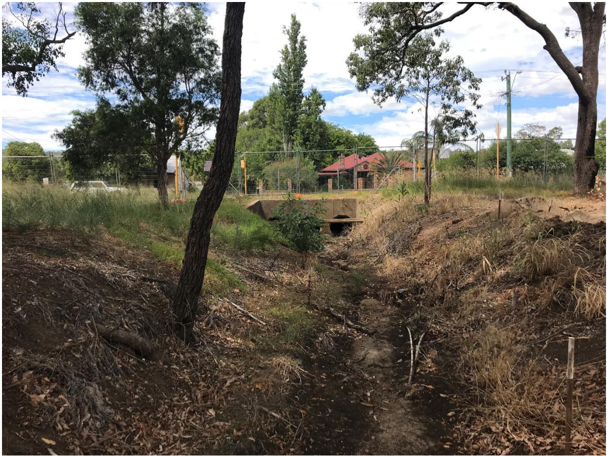
Structure No 30: Site 1.15 – Oaklands Drain at South Western Highway
