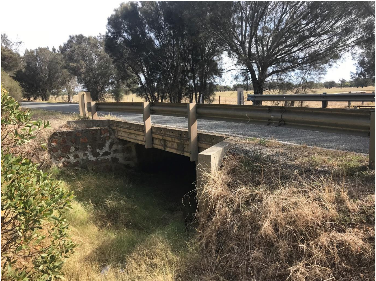
Structure No 83: Site 1.12 – Birrega Subdrain at Kargotich Road
