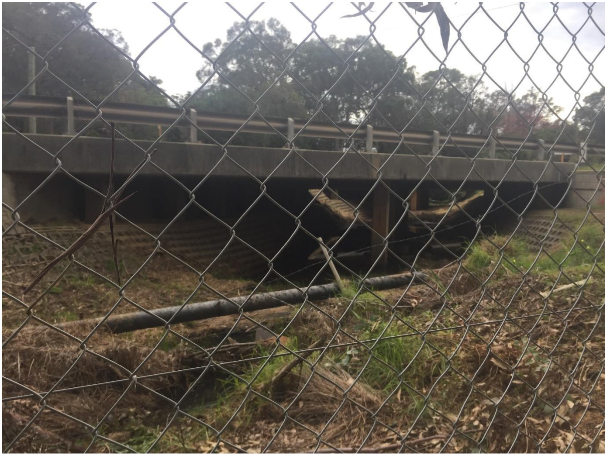
Structure No 39: Site 1.2 – Beenyup Brook at South West Highway
