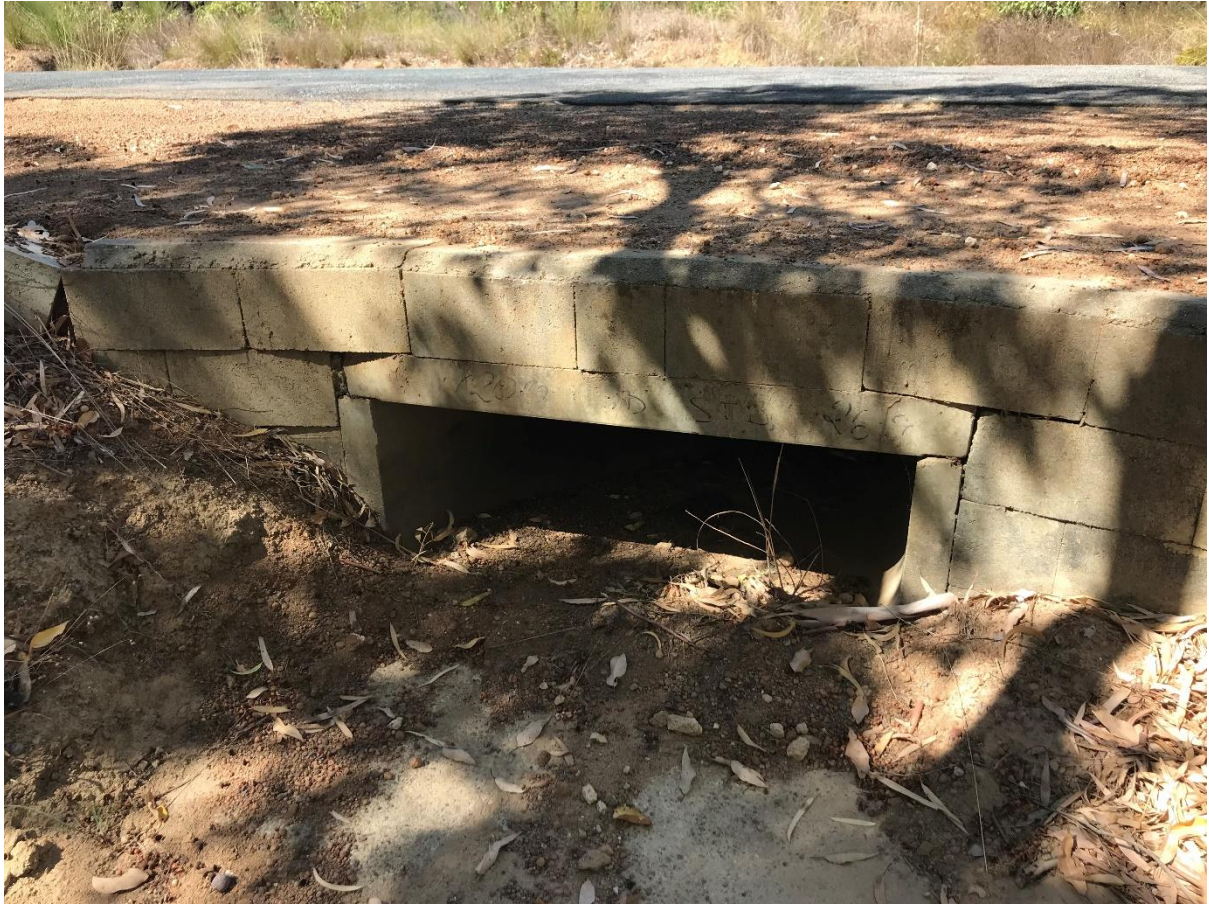
Structure No 56: Site 1.20 – Glades Multiple Use Corridor at Warrington Road
