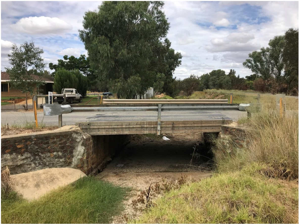
Structure No 51: Site 1.8 – Oaklands Drain at Abernethy Road
