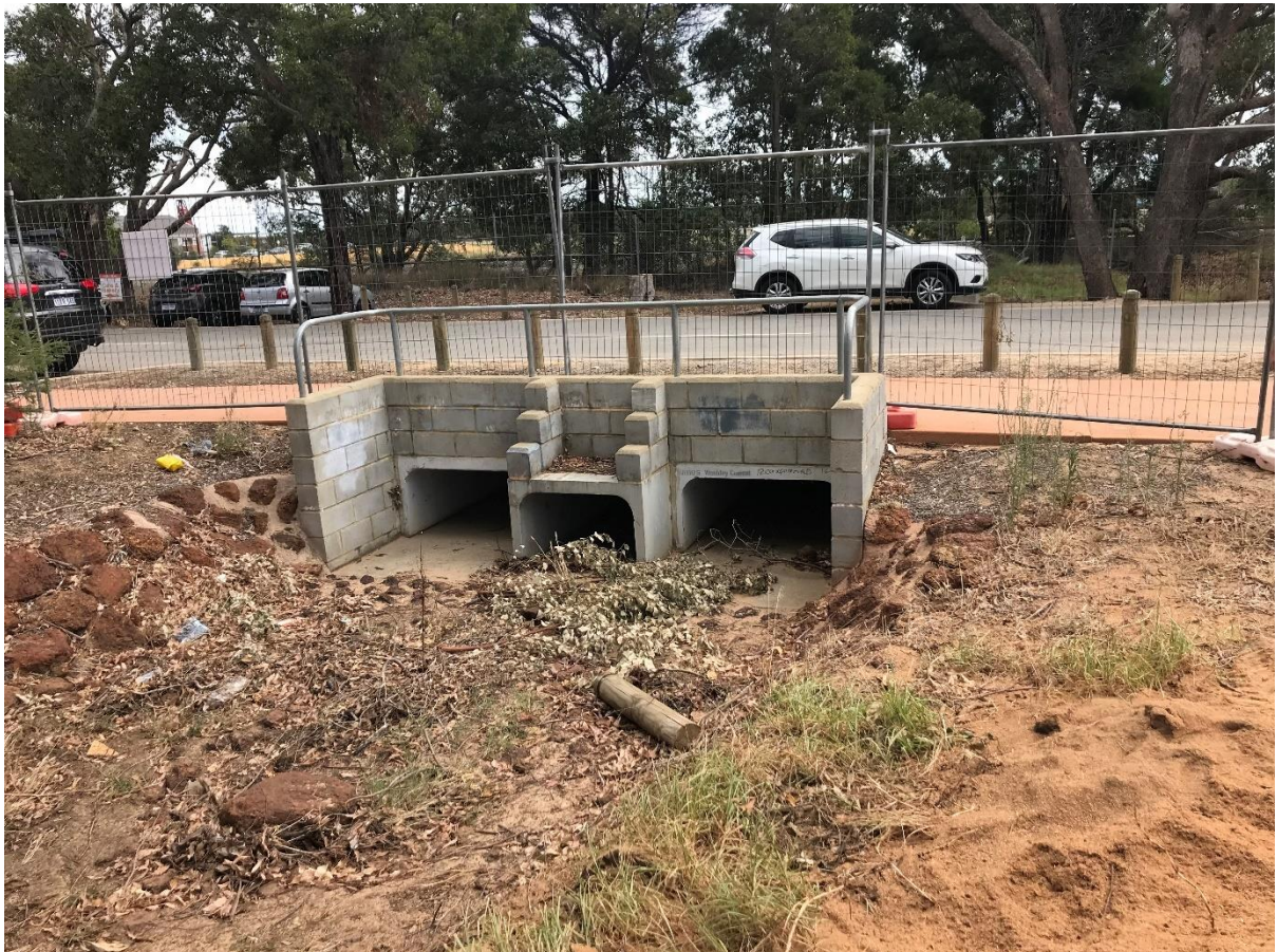
Structure No 30a: Site 1.15 – Oaklands Drain at George Street
