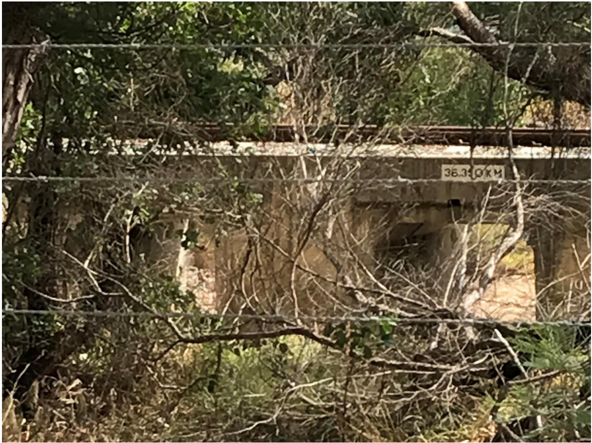
Structure No 31: Site 1.15 – Oaklands Drain at Railway
