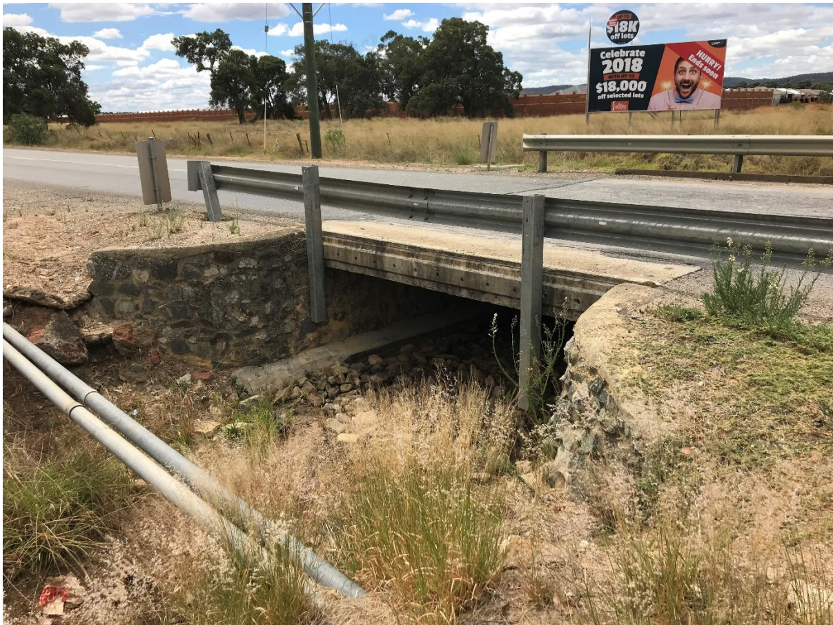
Structure No 49: Site 1.24 – Beenyup Brook at Hopkinson Road
