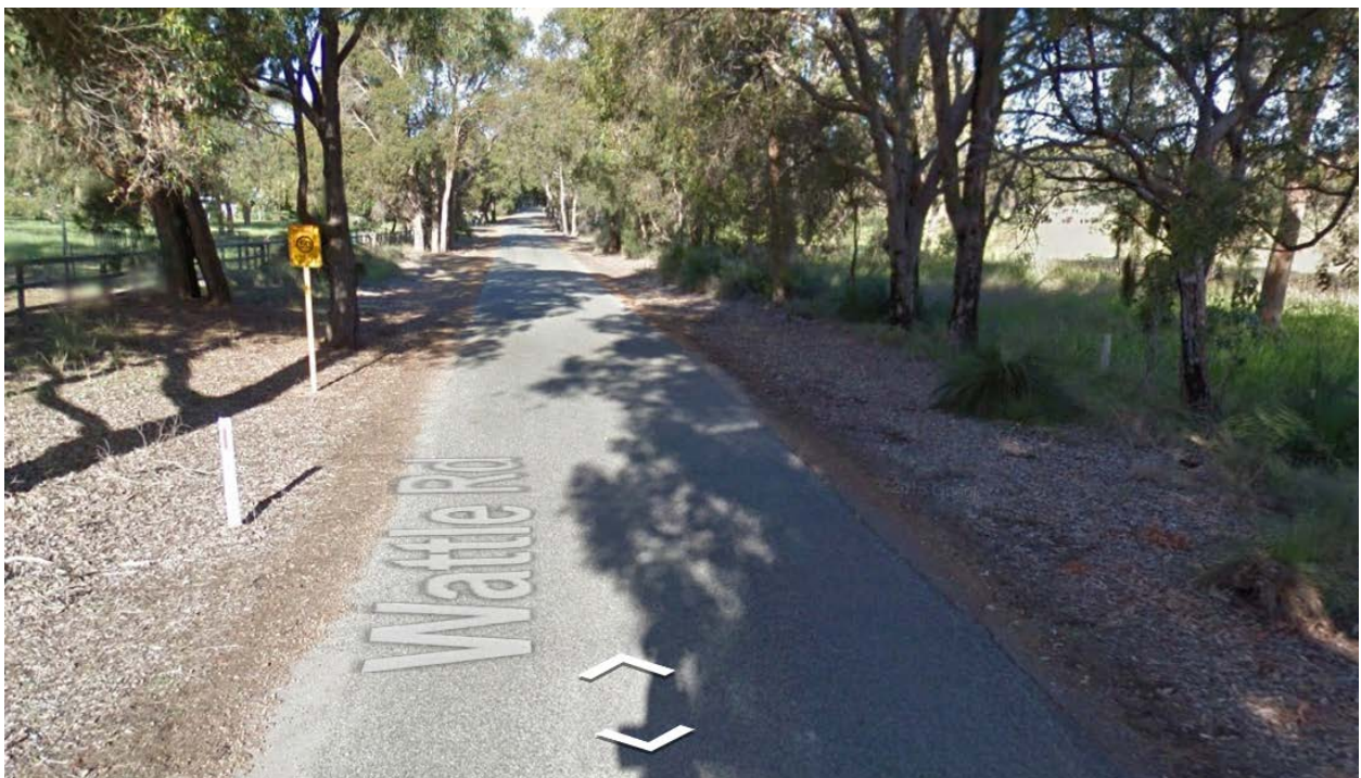
Figure 6. Wattle Road, looking east away from its intersection with Walker Road
