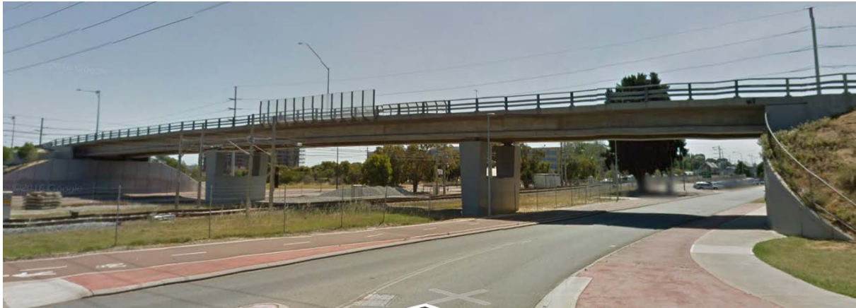
Figure 2-1 Road over Rail Crossing at Sevenoaks St & Railway Parade
