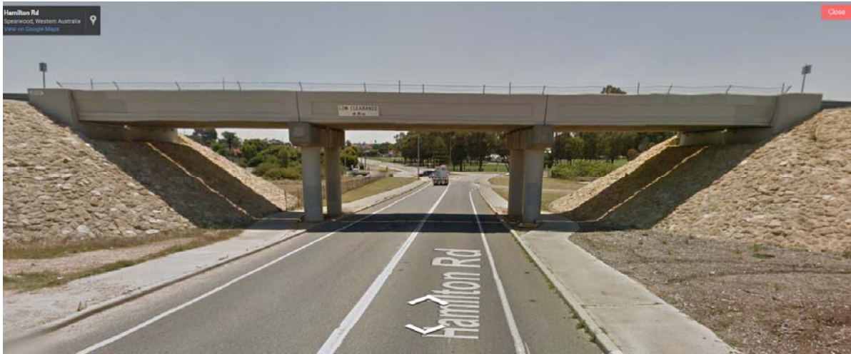
Figure 2-5 Rail over Road crossing at Hamilton Rd in Spearwood
