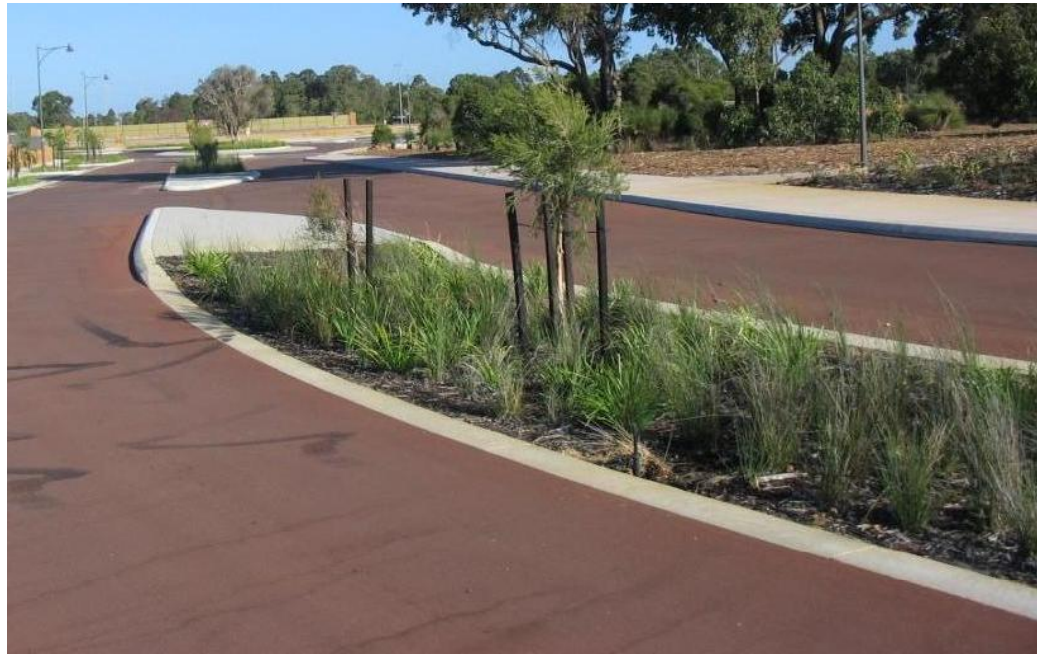
PHOTO OF TYPICAL VEGETATED SWALE TREATMENT
