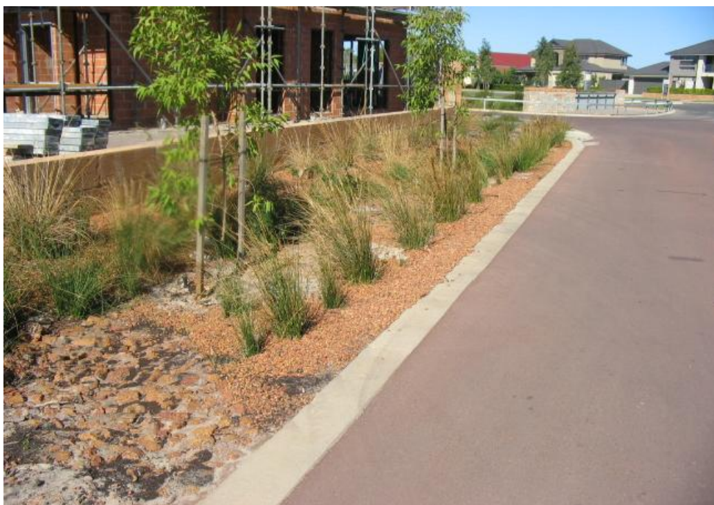
PHOTO EXAMPLE OF VERGE PLANTED SWALE
