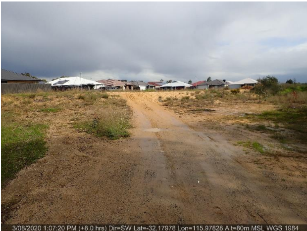
Photo ID: Photo 1 Looking at the cleared site ready for the subdivision.
