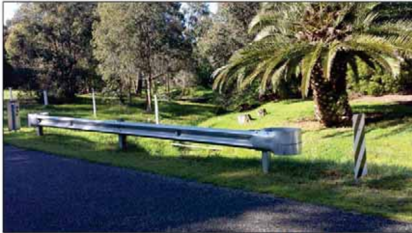
Photo 4 - Oaklands Drain crossing Stanley Road
