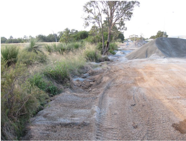
Area 5, view north
