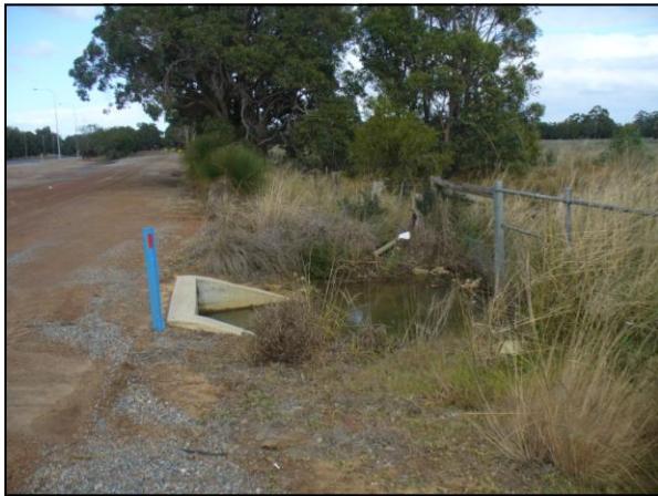
Existing drainage culvert from South Western Highway drain into drainage reserve between Lots 3 and 128.
