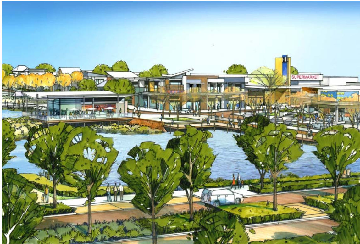
View south-east through the Village Centre
