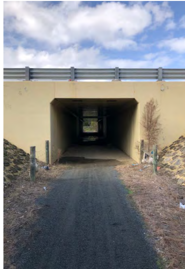
Figure 28 ▲ Existing Tonkin Highway equestrian underpass north of Thomas Road
