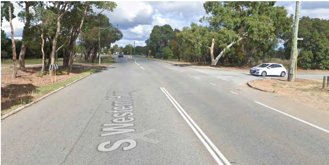
Figure 5: South Western Highway looking south at Larsen Road intersection
