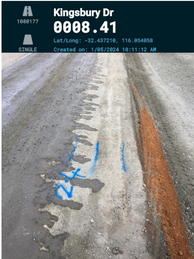
Image 3 - Rock in the swale location, with proposed kerb line in red:
