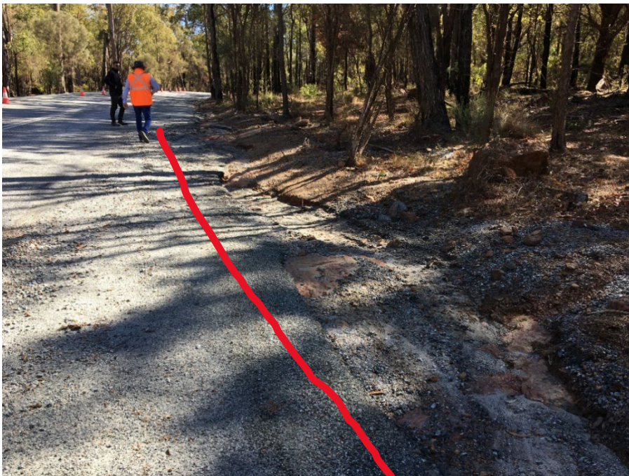
Image 3 - Rock in the swale location, with proposed kerb line in red:
