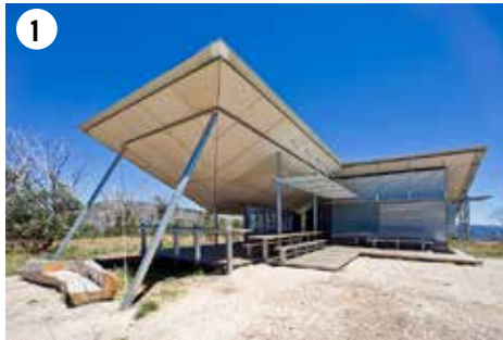
1 Multi-use 'signature' shelter that resides as an architectural statement in the landscape providing sense of place and Trails Head identity.
