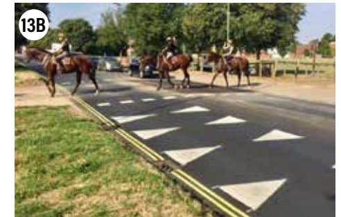
Horse and trail user crossing - gives presence to Trails Head location, provides awareness and slow down markers.
