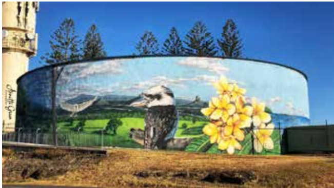
FIGURE 29. ARTWORK ON TANKS
