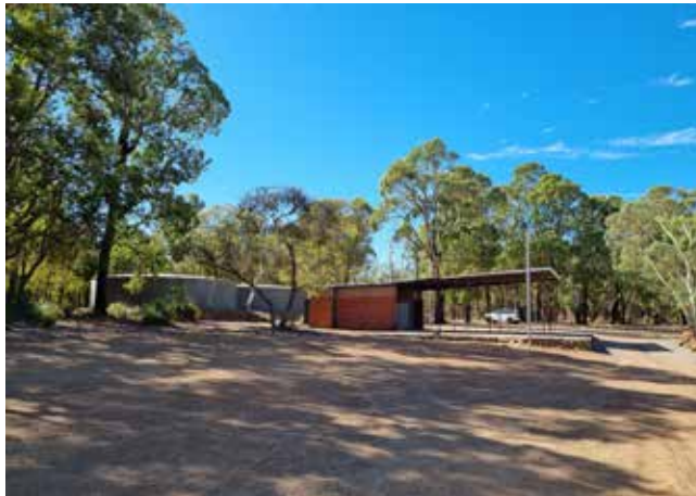
Looking north east towards the existing ablution block, DFES tanks and vehicle parking.
