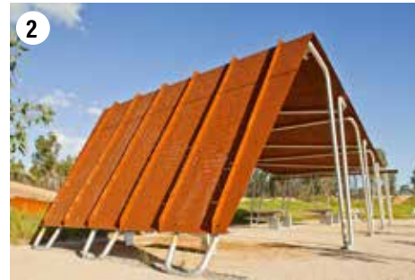
2 Trail head shelter - a basic muster point to gather and prepare before heading off to the many different trails. Wayfinding, seating and water.
