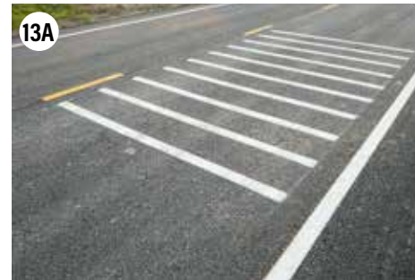
Traffic calming devices to reduce vehicle speed and driver awareness of trail users crossing.
