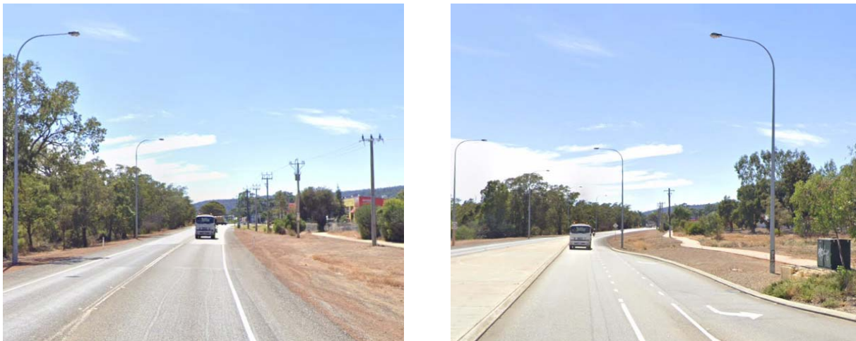
Figure 3 – South Western Highway
