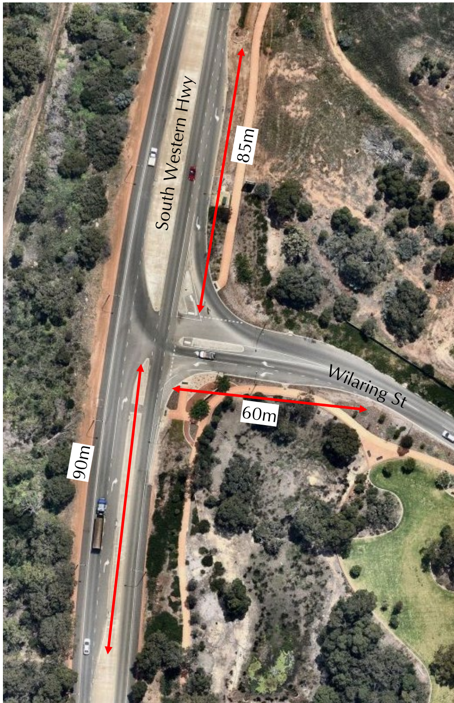
Figure 5: Existing standard of the intersection of SWH/ Wilaring St
