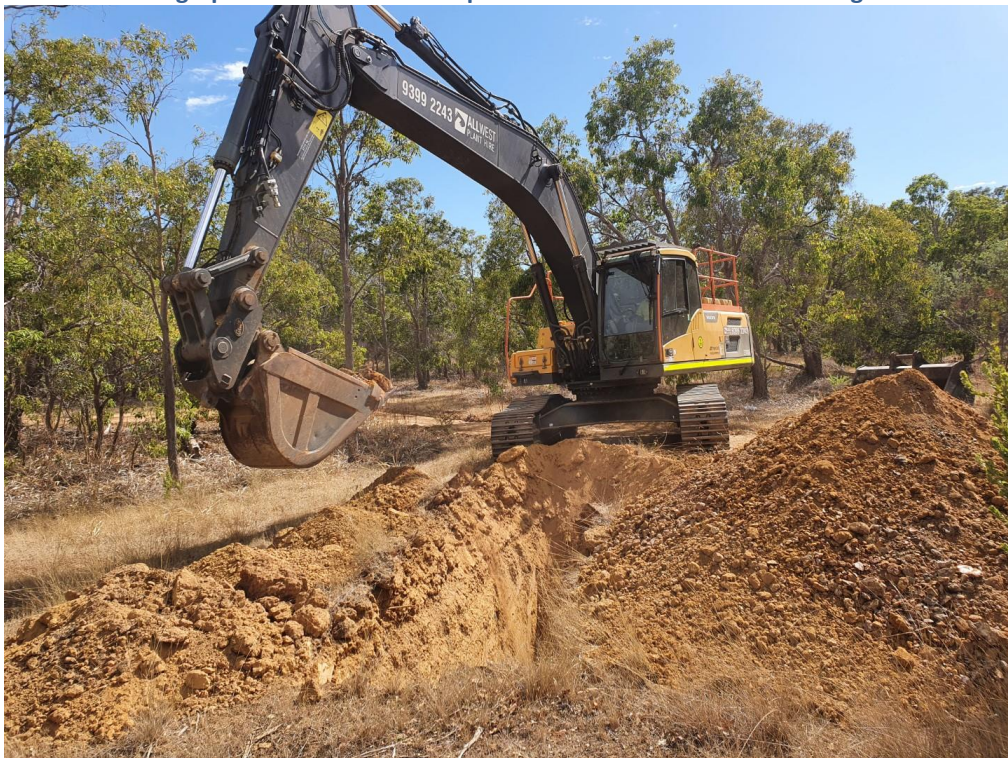
Photograph 4: View of test pit excavation (TP21) Ordinary Council Meeting - 17 June 2024
