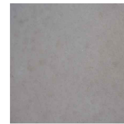
6 PORTLAND PRECAST CONCRETE PANELS
