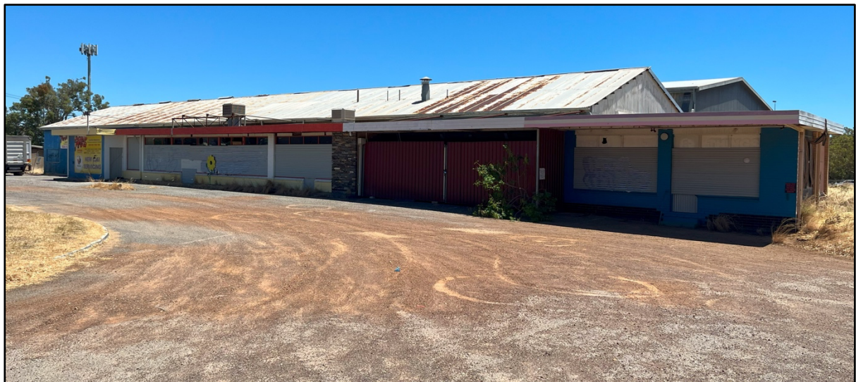
Photograph 1 - Existing development on the subject site, looking south-west.
