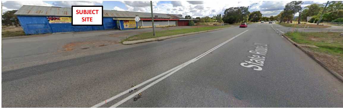
Figure 4. Northbound view along South Western Highway
