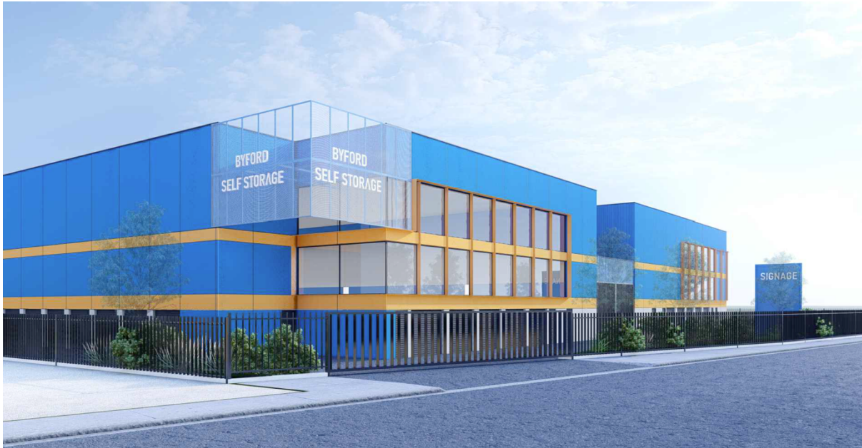
Figure 4 - Development, as viewed from South Western Highway.
