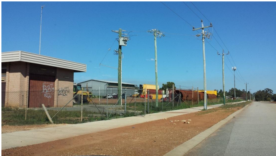
View of existing Transport Depot from western boundary facing south
